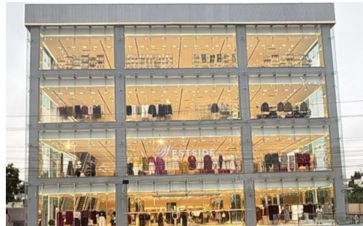
SNB Tower, Udaipur
